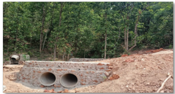
Humpe Pipe Culvert To Channelise Water
