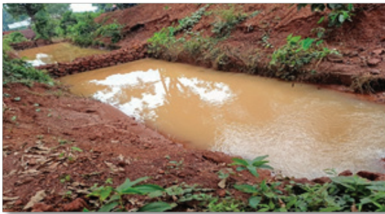
Series Of Gully Plugs To Control Erosions
