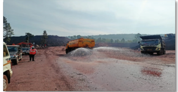
Haul Roads Dust Suppression
