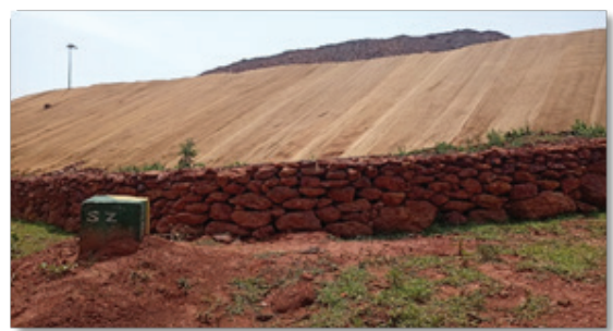
Coir Matting & Rubble Wall For Waste Dump
